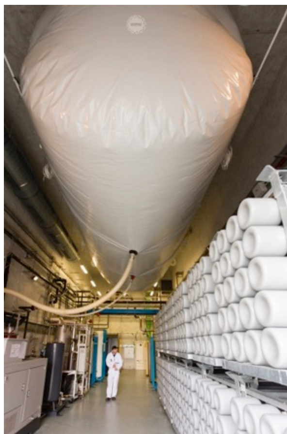
Cryogenic plant where liquid helium is produced for the Spiral2 Linac (LINear ACcelerator). © Philippe Stroppa/CEA/CNRS
