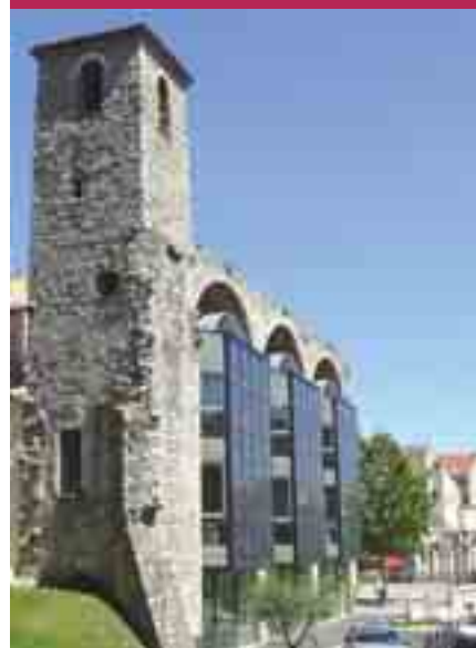
A unique example of the use of the double-skin concept with an integrated photovoltaic device at the Cévennes Tourist Office.
