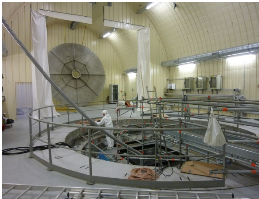
Overview of the second detector with, in the foreground, the mouth of the detector tank before the installation of its cover.
