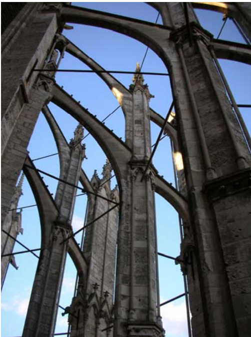
Steel tie-rods between the flying buttresses of Beauvais cathedral.
